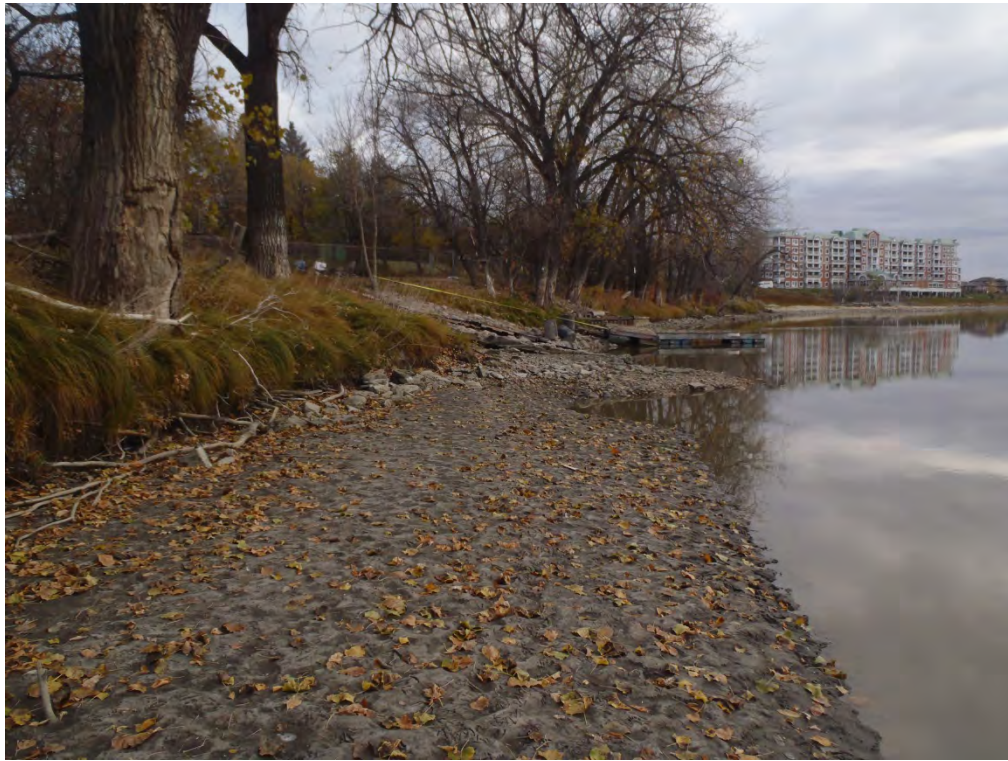
Figure 04: West Riverbank (October 23, 2013)
